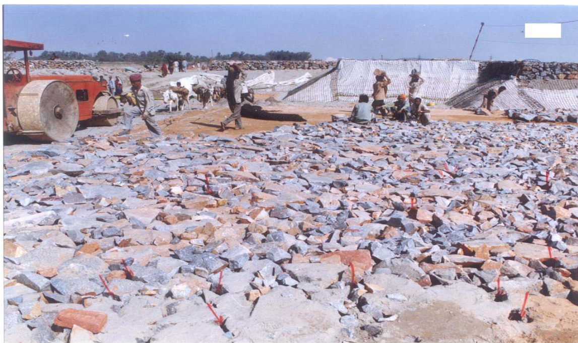
Fig.6(b). Photo plate showing the geo fabric, overlaying rope mattress and stone
