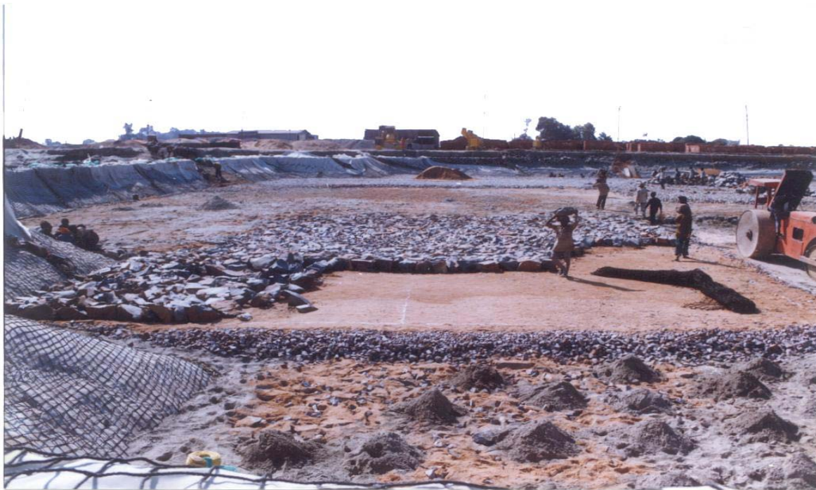
Fig.6(a). Sequential construction of the foundation system shown in fig 5 in a typical cross section
