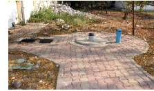
(b) Furaat System with Water Meter Chamber and Recharge Bore
