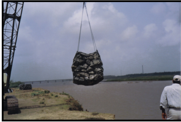
Fig.2: Rope Gabbion laying under water on riverbank at Umra, Surat
