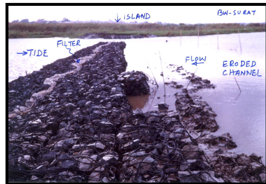
Fig. 8: Laying of Gabbions, Filter in stages in tidal zone.
