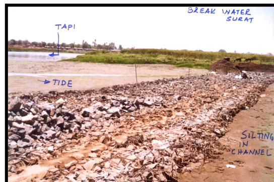
Fig.10: Silting on Weir & Island side (2000).
