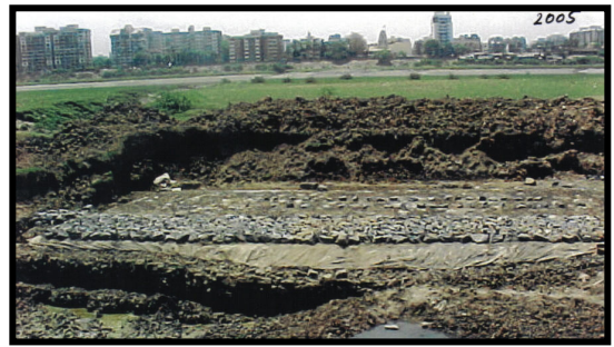
Fig. 20: Finalized profile protection against erosion at Surat.
