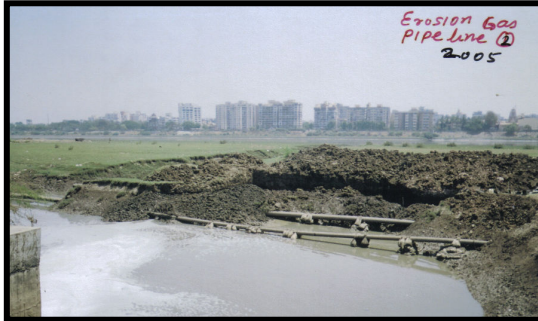
Fig. 17: Gas Pipeline Bed Erosion, Pal, Surat.
