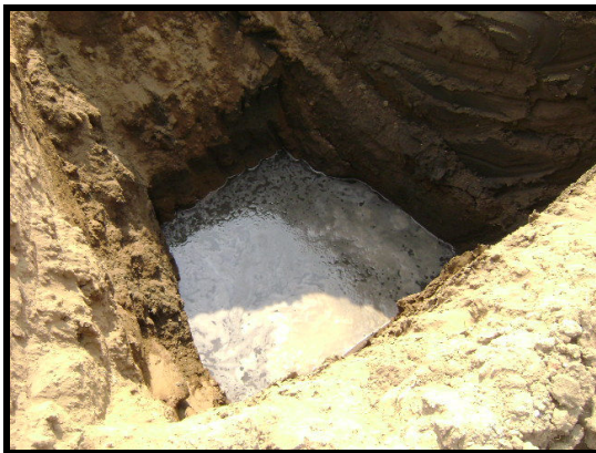
Fig. 32: Ground water seepage at foundation level after excavation at SIECC Sarsana.
