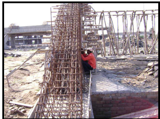
Fig. 35: Foundation above ground level on treated soil at SIECC.
