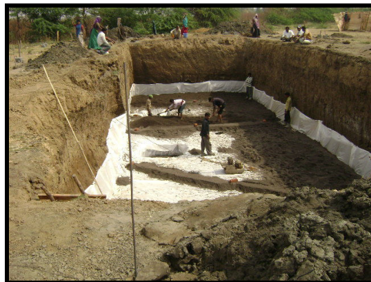
Fig. 34: Proving Sand layer above Geotextile at SIECC.
