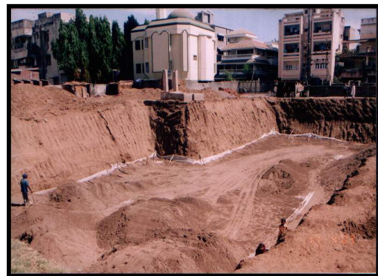
Fig. 29: Providing fabric & fill & compacting in layers
