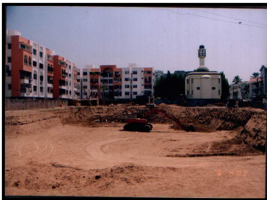
Fig. 28: Excavation of Creek zone at ABRAR apartment.
