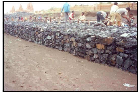
Fig. 14: Final layout, backfill with Sand at BAPS, Tithal.
