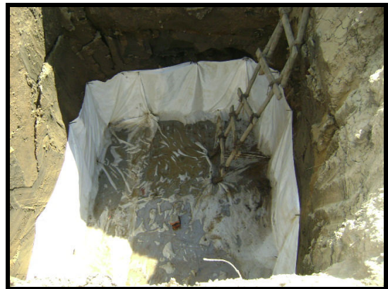
Fig. 33: Laying of Geotextile at foundation level for SIECC.
