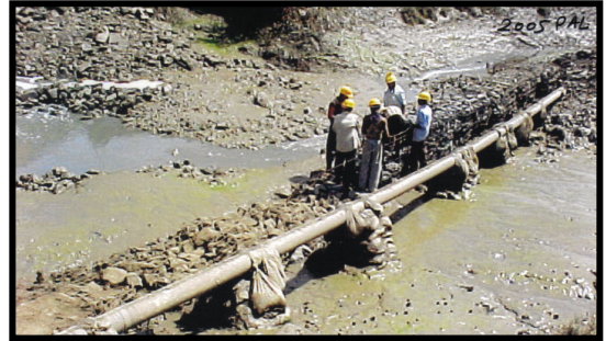
Fig. 18: Erosion protection treatment by Gabion & Geo-filer: Geo-synthetics.
